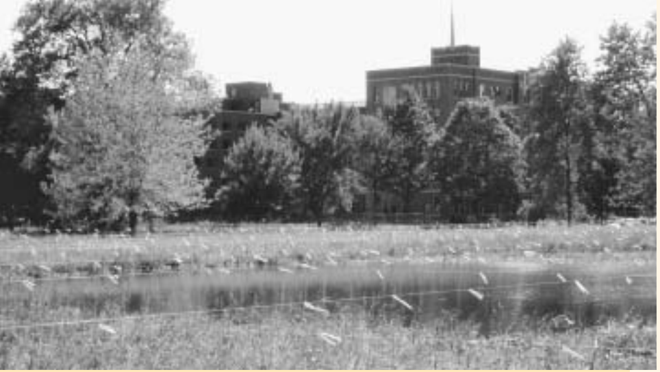
As part of the greywater system, grey water goes to this constructed wetland for natural treatment before returning to the Motherhouse for flushing toilets. The plantings are part of the cleansing process.
