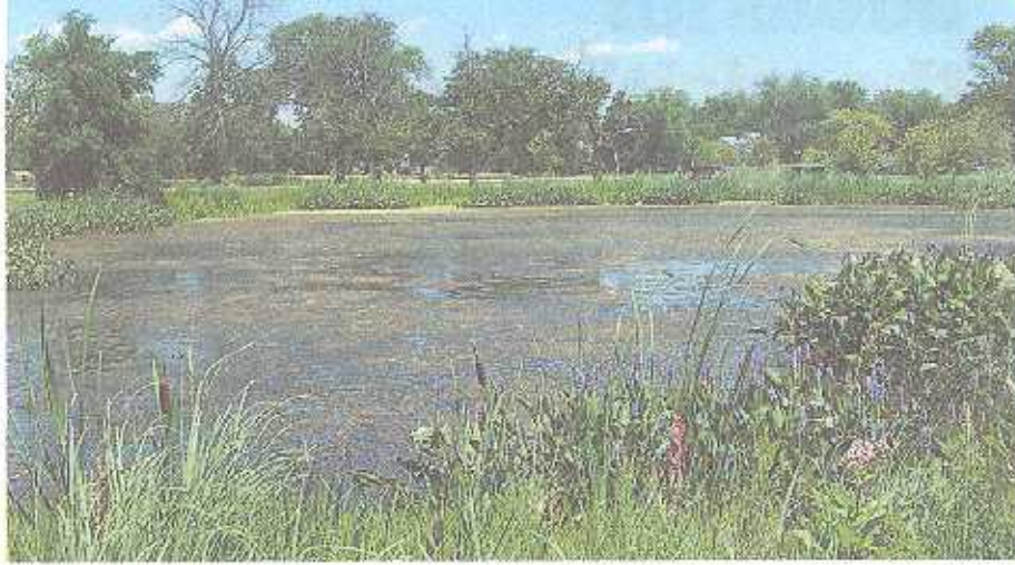
The manufactured pond filters sink and bath water through special vegetation and pea rock to return it as clear water for the facility's toilets.
